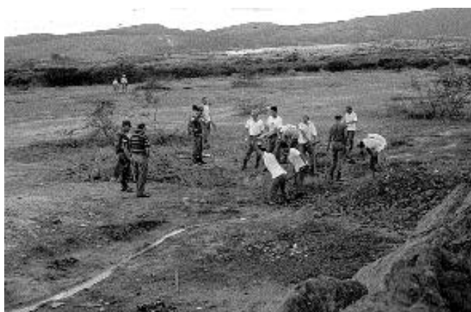
First excavations at the landing strip of the Vallegrande airport, December 1995
